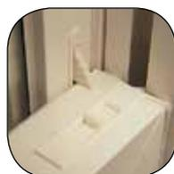
Vent locks allow for partial opening of sashes. Tilt latches allow easy tilting for cleaning.
